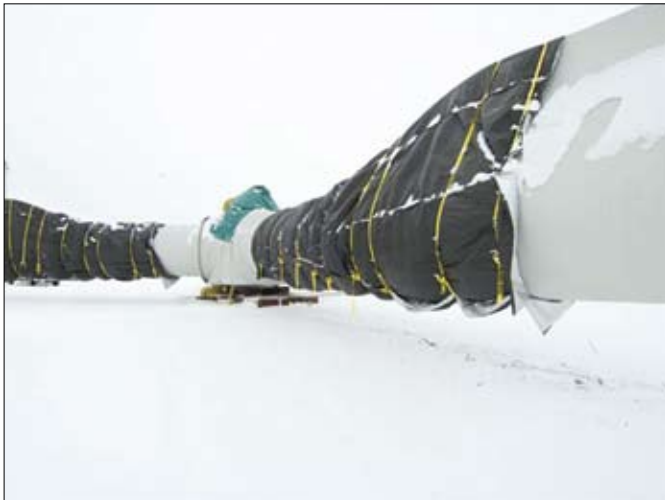
Rotor with thermal insulation wrap to facilitate curing of laminate during blade reinforcement
